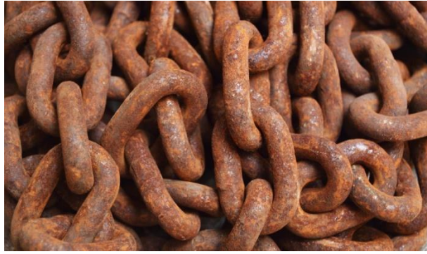
Figure: Uniform Corrosion
